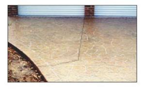
Figure 3: Joint perpendicular to slab edge
